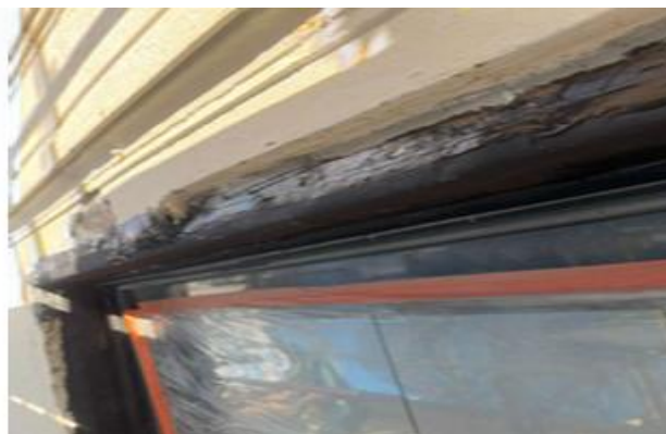
Ongoing EPDM Installation
