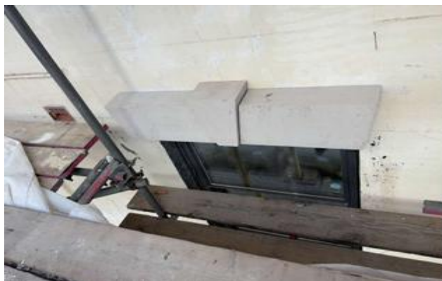
New Head Stonework Installed
