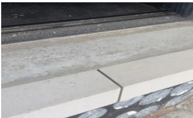
Completed Stone Cill & Concrete repair
