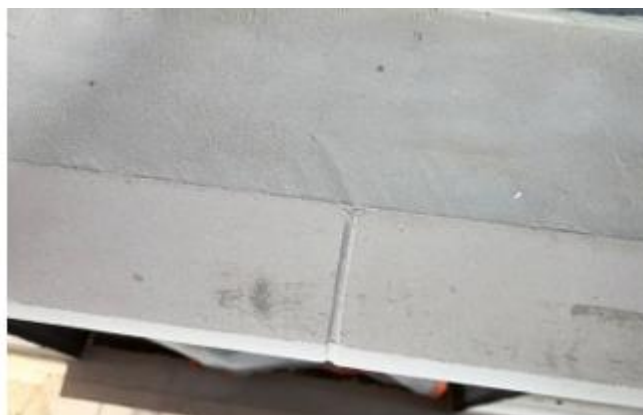
Completed Stone Cill & Concrete repair
